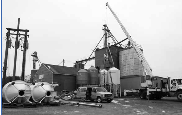
Workers install two 16-ton bins to hold finished feeds.
